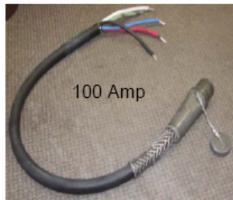
Figure D- 3 100 Amp per Phase Feeder System - 3 Phase
