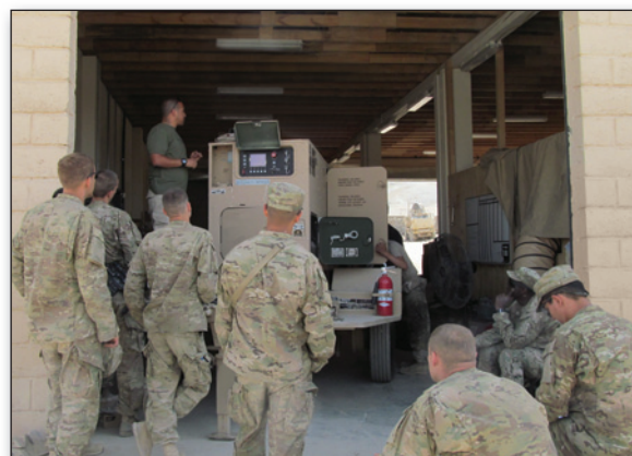
U.S. Army troops in Afghanistan receiving training on a trailer-mounted AMMPS unit.
