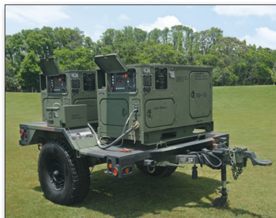
Photo credit: U.S. Army. Two AMMPS units mounted on a trailer. Paralleling them is easy.
