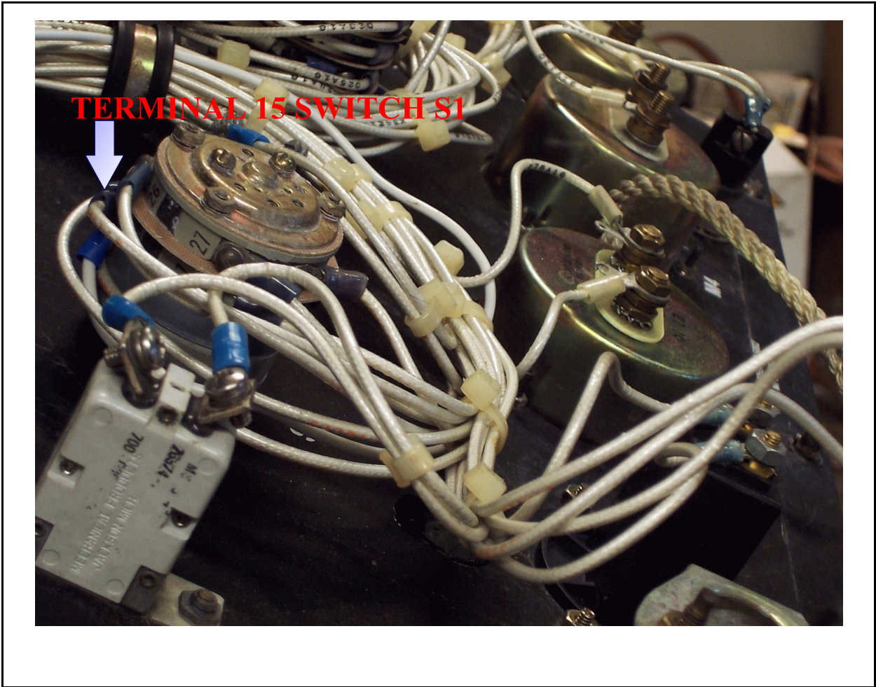
This concludes the wiring of the Circuit Board with the Generator Set itself.
