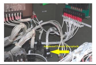
The first Amphenol Receptacle is mounted in the bottom of the Control Cubicle and wired with the Auto Starter PCB
