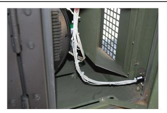
The Connector connects to the Receptacle on the bottom of the Control Cubicle and has an other receptacle on the other end mounted on the side wall of the unit
