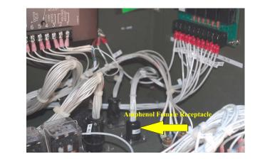
The first Amphenol Receptacle is mounted in the bottom of the Control Cubicle and wired with the Auto Starter PCB
